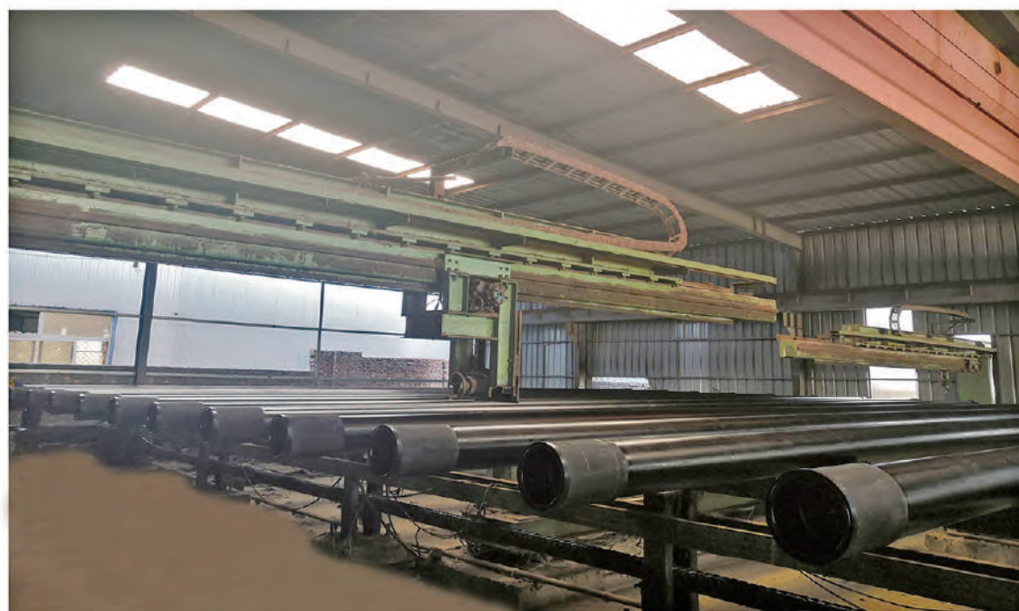
测量承重设备 / Measuring load-bearing equipment
